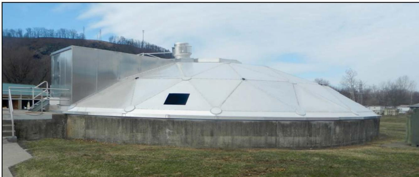
***WATER PLANT RENOVATED CLARIFIER WITH ALUMINUM DOME COVER***
